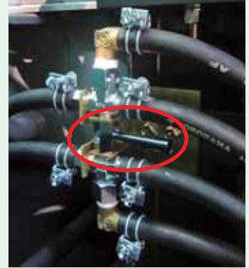
▲ Changeover cock of fuel tank
