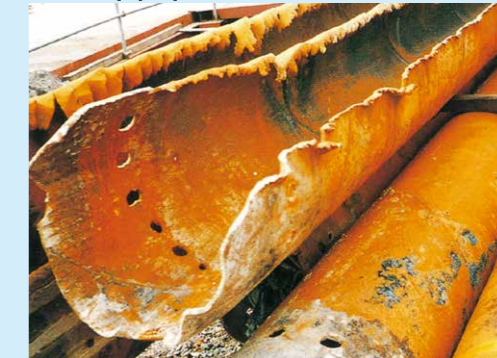
▼ Steel pipe pile.
