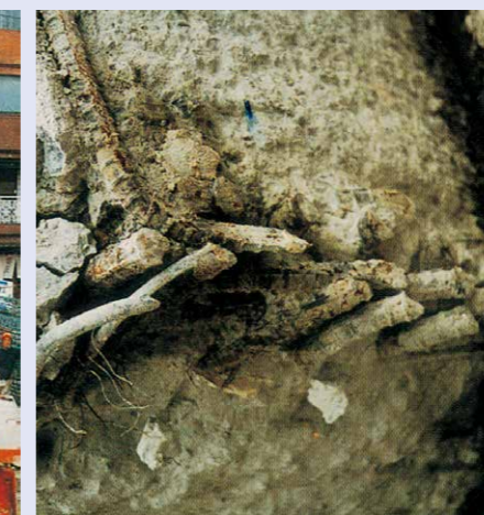
▲ Reinforced concrete foundation.
