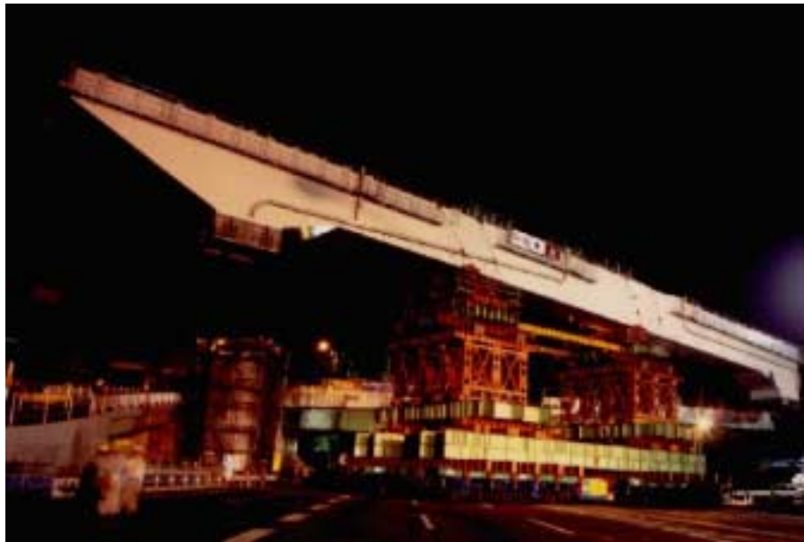
Nagoya Minami IC (under construction) and heavy-duty carrier
