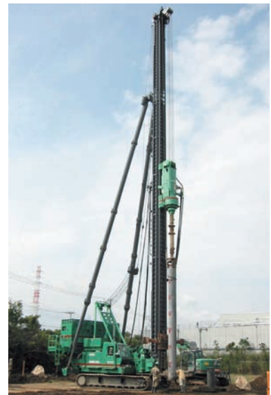
Pile Driving Rigs
