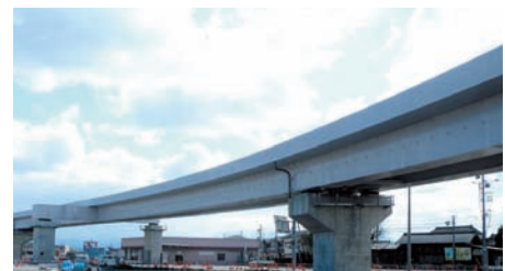
the Shibata Elevated Bridge
