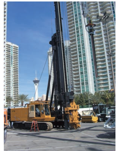
Pile Driving Rigs
