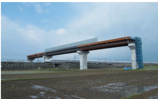
the Kozakai Bo Bridge
