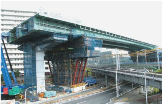
Construction Project of Otobashi overbridge
