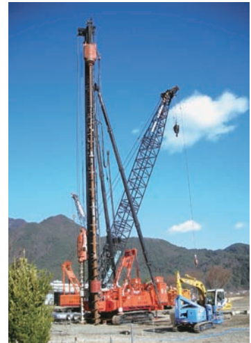
Pile Driving Rig
