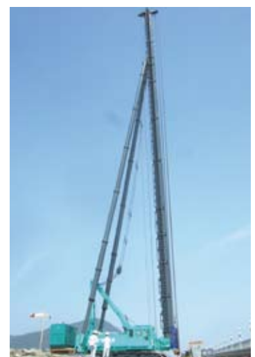
Pile Driving Rig
