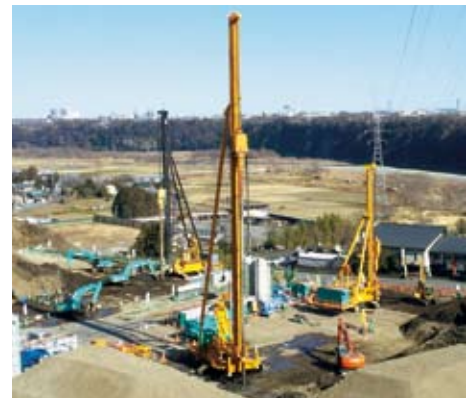
Large Pile Driving Rig
