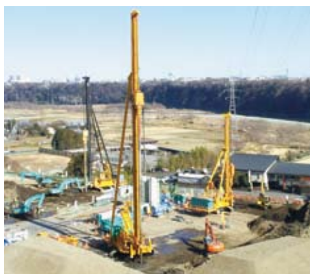
Large Pile Driving Rig
