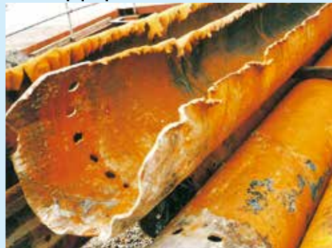
▼ Steel pipe pile.
