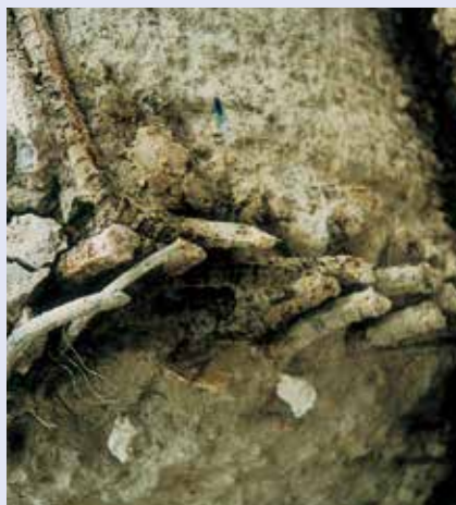
▲ Reinforced concrete foundation.
