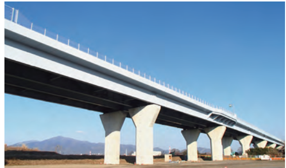
Miyayama Elevated Bridge
