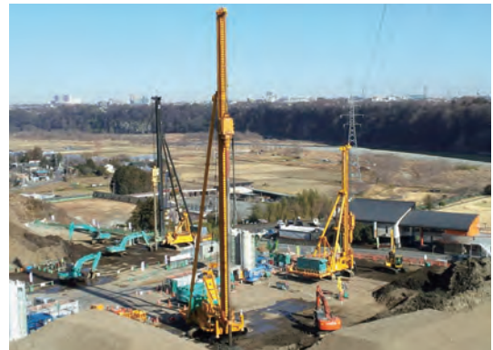
Large Pile Driving Rig
