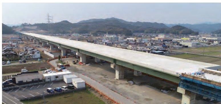
Tokai-Kanjo Expressway Nagafuke Number 4 Bridge
