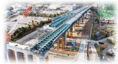
Shin-Komakado-Higashi Number 3 Viaduct
